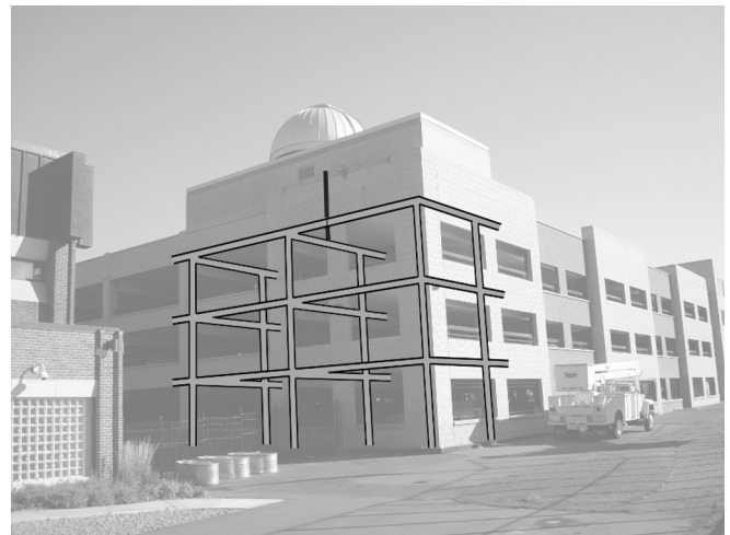
Fig. 1. A schematic view of the support structure underneath the telescope pier. The pier is attached to a crossbeam between two concrete columns extending to the building foundation. This structure shields the telescope from oscillations in the parking deck.
